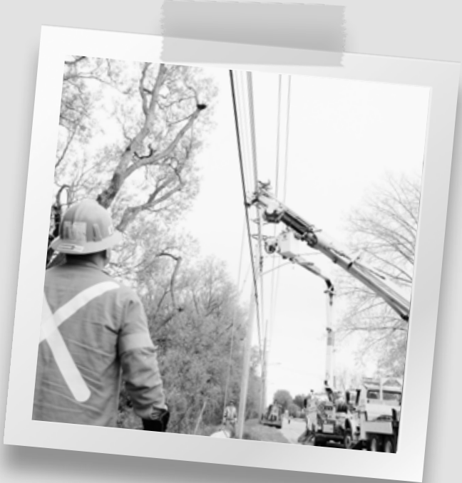
POLE UPGRADES IN COLBORNE
